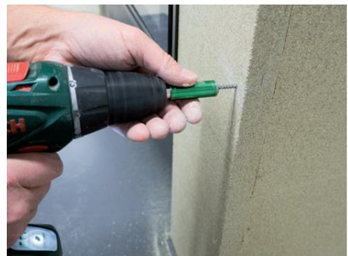
Build individual dream fireplaces with **THERMAX® SN 500** fireplace construction boards. Use standard woodworking tools to machine the boards. The boards are bonded together with adhesive and can also be screwed together without pre-drilling.
